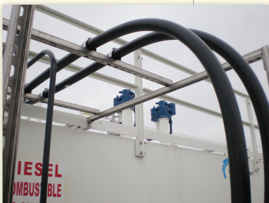
US Navy specified a ten thousand gallon AST of which 7000 was for Gasoline and 3000 for Diesel. (DoubleTrac pictured above)
